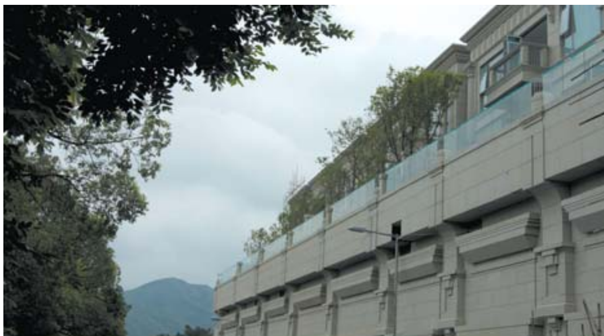
Proposed residential redevelopment of Yucca de Lac, Shatin — Design, supply and installation of aluminium window and “Schüco” folding door 沙田雍雅山房的建議住宅項目—設計、供應及安裝鋁窗及「旭格」摺門
