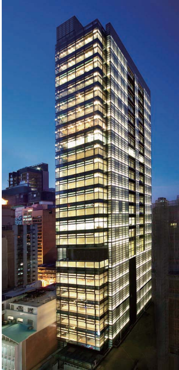
Construction of The Cameron at 33 Cameron Road, Tsim Sha Tsui 興建位於尖沙咀金馬倫道33號之The Cameron
