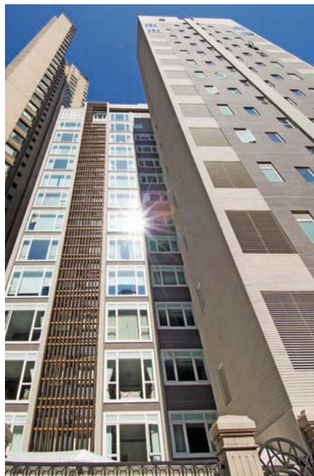
Alternation and renovation works for Tavistock at 10 Tregunter Path in Mid-levels 半山地利根德里10號騰皇居的改建及維修工程
