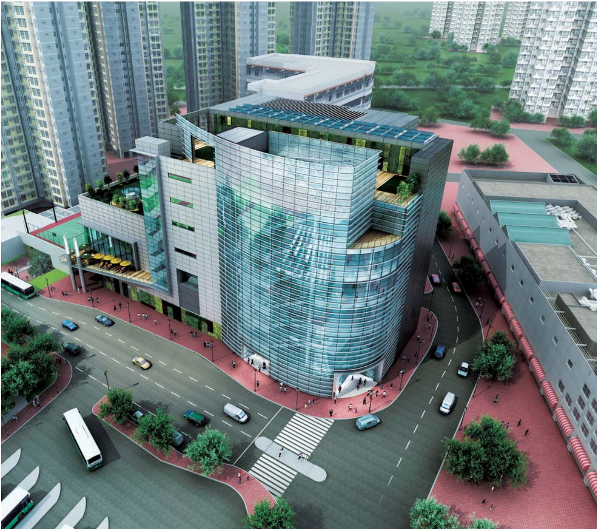
Construction of Lam Tin North Municipal Services Building 興建藍田北市政大樓
