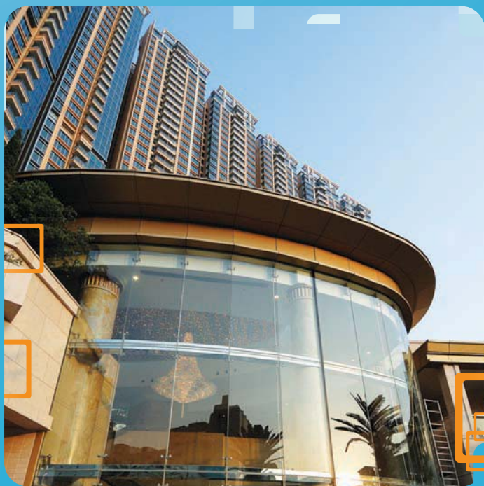
The Palazzo at 28 Lok King Street in Shatin — Design, supply and installation of glass walls 沙田樂景街28號御龍山 — 設計、供應及安裝玻璃牆
