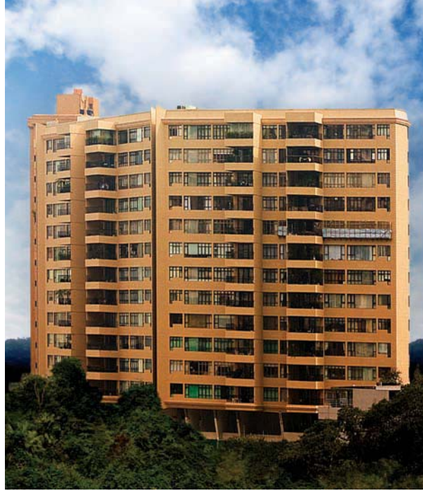
Refurbishment, renovation and alternation works at Grenville House at 1-3 Magazine Gap Road, Mid-levels 半山馬己仙峽道1-3號嘉慧園的翻新、維修及改建工程
