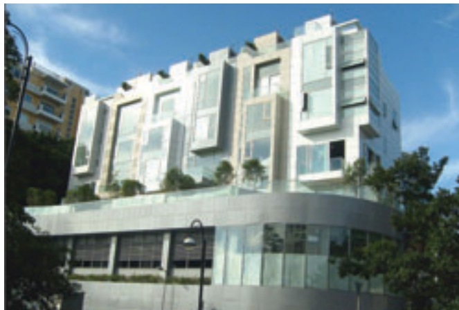
Design, supply and installation of "Schüco" windows, curtain walls, louvres, external metal and stone claddings for the residential development at 3-5 Plunkett's Road in The Peak 為山頂寶吉道3-5號住宅發展項目設計、供應及安裝「旭格」鋁門窗、幕牆、百葉、外牆金屬及雲石飾板
