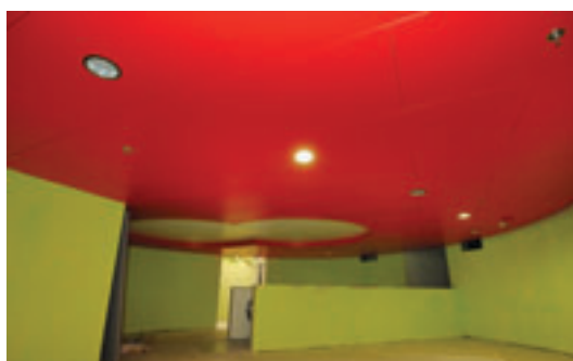
Supply and installation of false ceiling at Chai Wan Youth Development Centre in Chai Wan 為位於柴灣之柴灣青年發展中心供應及安裝假天花
