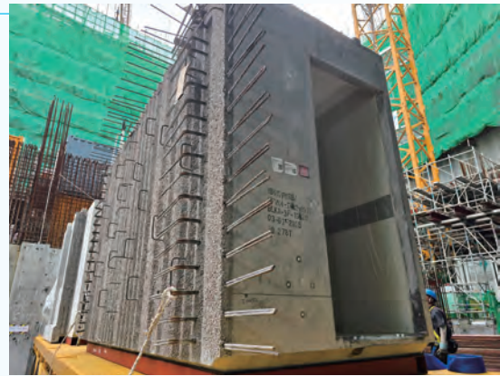
Delivery of VPK to the construction site
