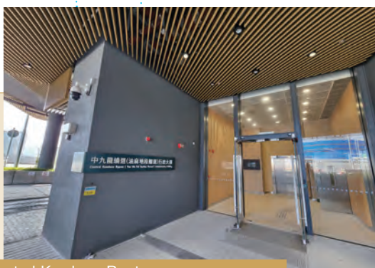
Central Kowloon Route – Building, electrical and mechanical works
