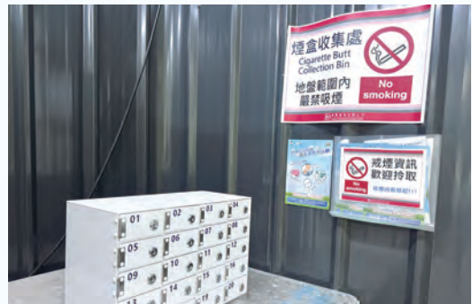
Placement of cigarette butt collection bin at the site entrance to reduce fire hazards and support a smoke-free workplace
