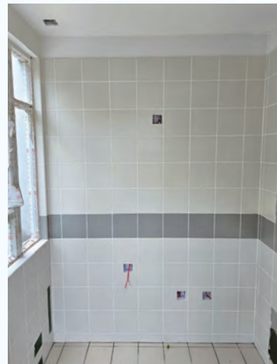
Interior fit-out of VPK
